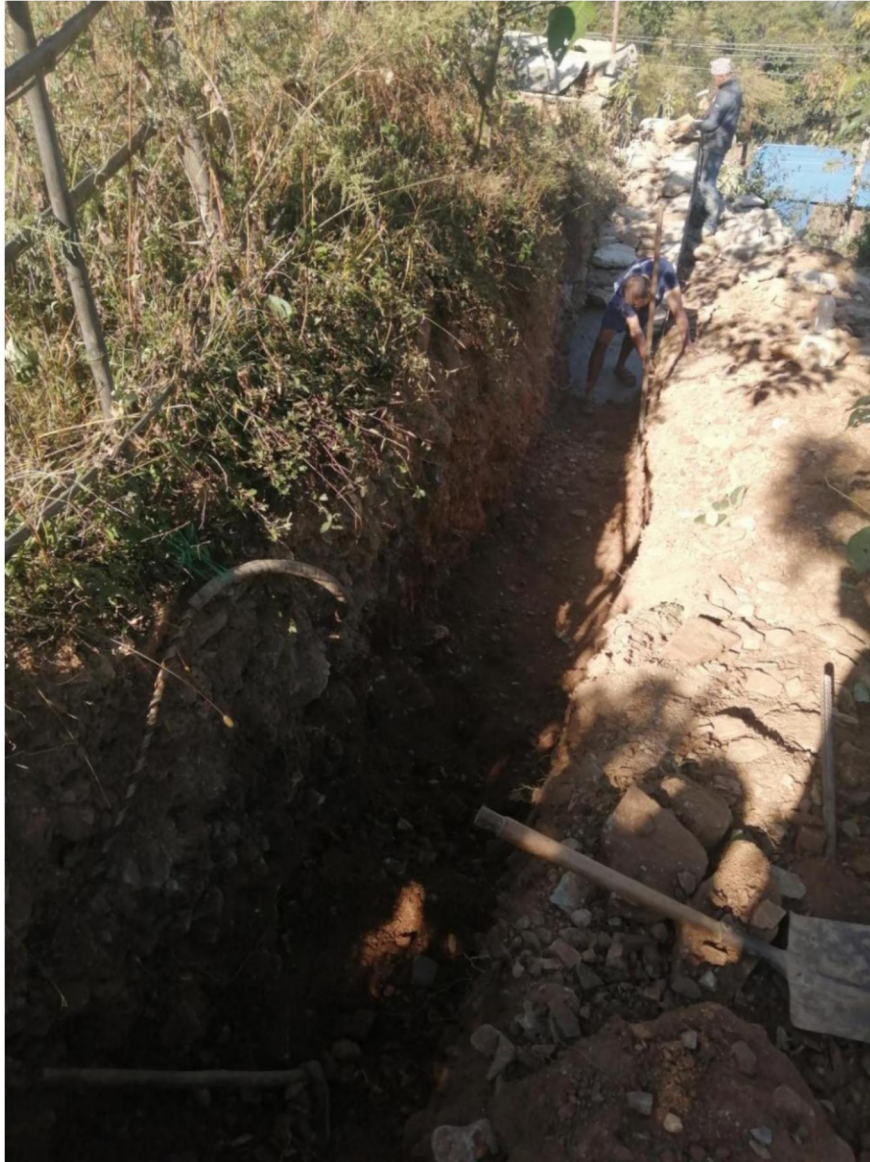
(Helping to dig out the trenches for laying the wall foundation)
