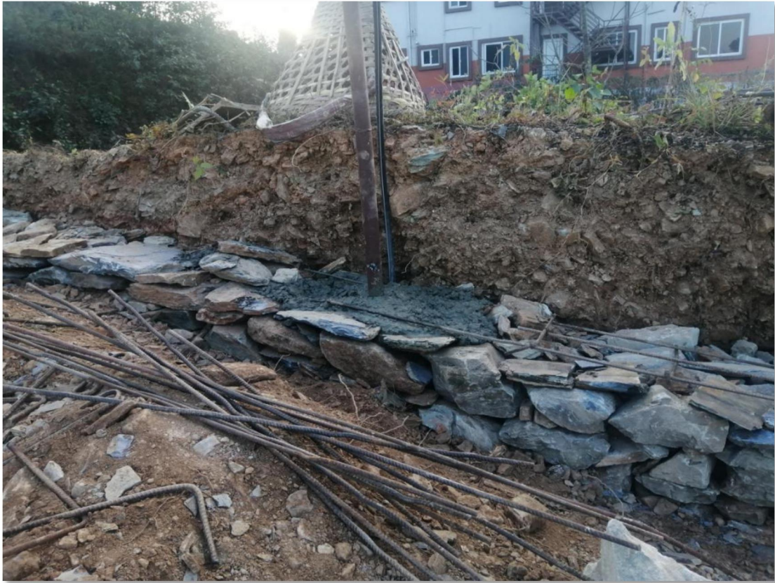
(Posts that are anchored within the wall for future fence installation and light application)
