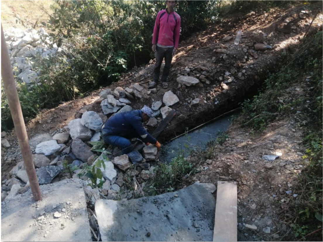
(Local mason applying the concrete mixture for the wall construction)
